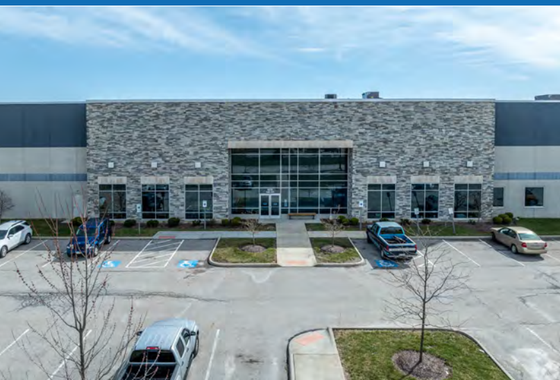
Main Building Entrance
