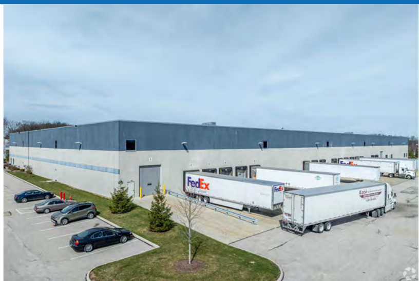
Exterior View: Drive-in Doors and Docks
